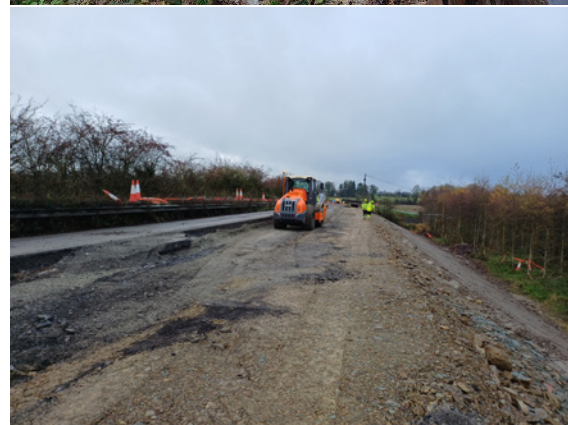
Construction of a widened embankment near Fowlard's Bridge on N55
